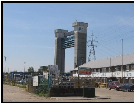
Barking Creek Flood Barrier
