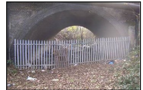
Tunnel under railway (L2)
