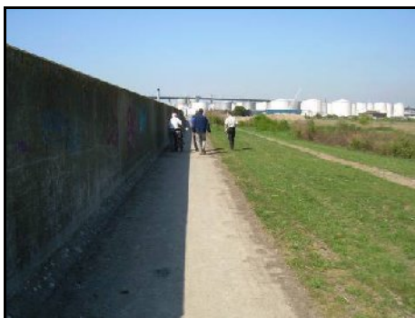
View towards QEII Bridge
