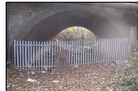
Tunnel under railway (L2)
