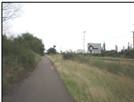
Existing shared use path set well back from the main road
