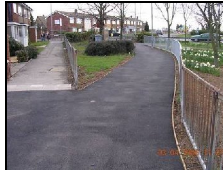
Shared path beside The Manorway within Stanford-le-Hope
