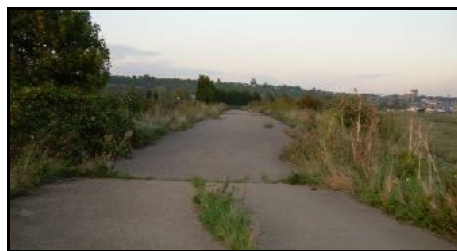
Existing concrete roadway
