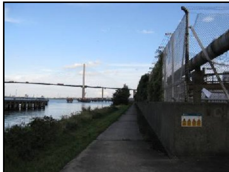
Littlebrook Power Station
