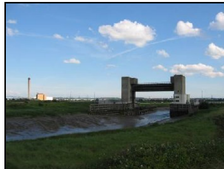
Dartford Creek Barrier
