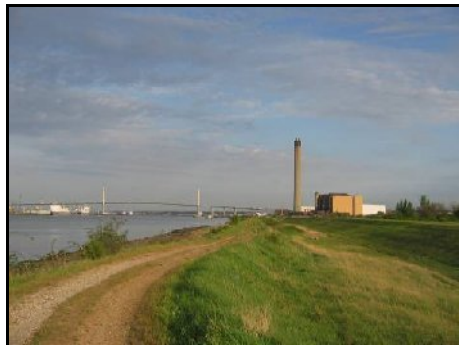
Looking east to QEII Bridge
