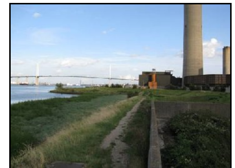
Littlebrook Power Station
