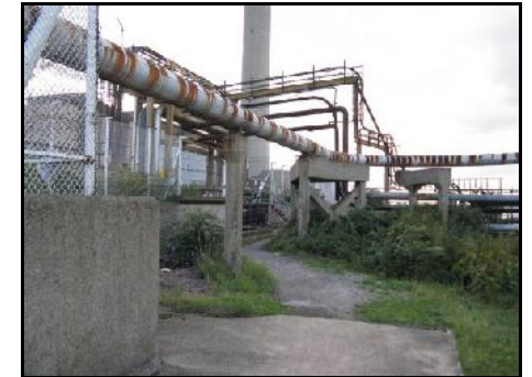
Jetty adjacent to power station
