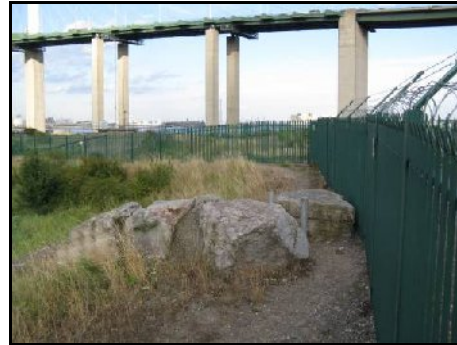
Access control above Dartford Tunnel
