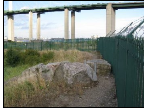
Access control above Dartford Tunnel
