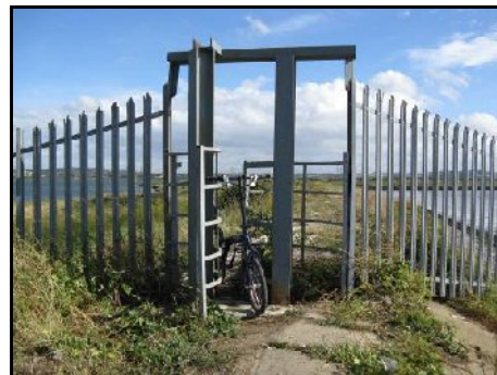
Access control at B2
