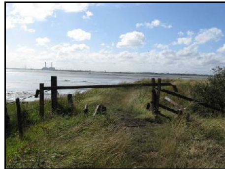
Metal barrier at B1
