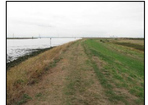
Flood defence embankment
