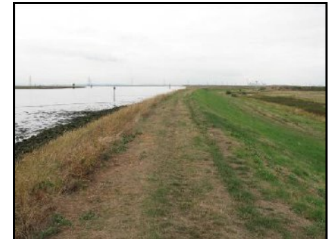
Flood defence embankment
