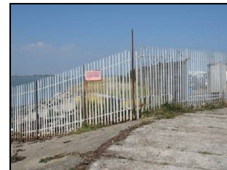
South end of car storage area
