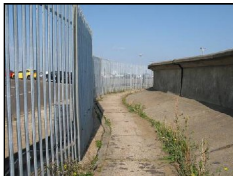
Sea defences beside car storage area
