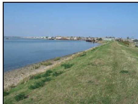
Looking north to Queenborough
