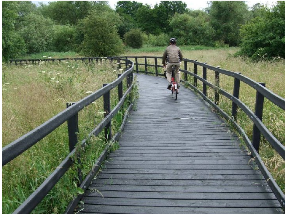
Plastic elevated walkway in Sutton Coldfield
