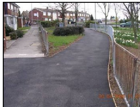
Shared path beside The Manorway within Stanford-le-Hope
