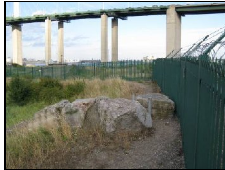
Access control above Dartford Tunnel
