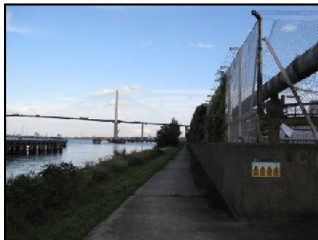
Littlebrook Power Station
