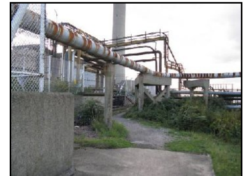
Jetty adjacent to power station
