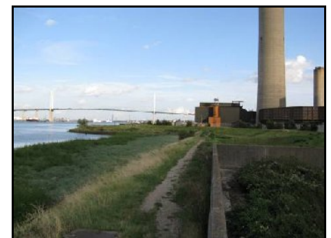
Littlebrook Power Station
