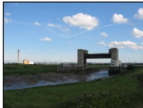
Dartford Creek Barrier
