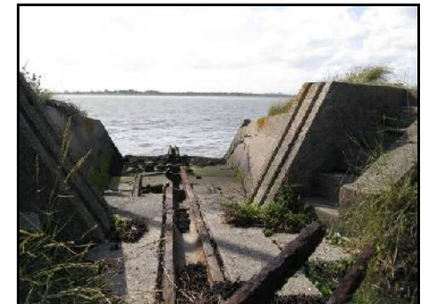
Torpedo launch tube at Cliffe Fort
