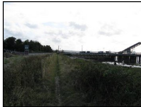
Jetty at Cliffe Fort
