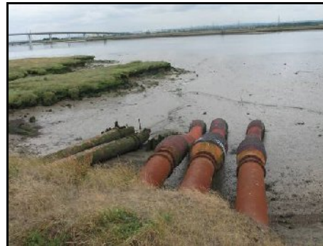
Sewage Works outfall pipes
